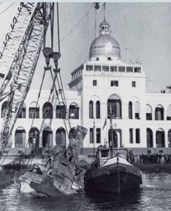
Cranes were used to lift the sunken obstacles in the Suez Canal.
