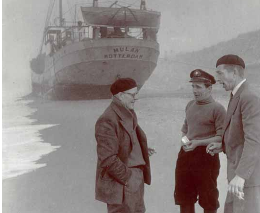
MULAN OF ROTTERDAM grounded at Thy, Denmark. The captain of the ship is in the middle of the group and the SVITZER captain P. Underlien on the right. The vessel was lifted by hydraulic jacks 20 metres into the sea to a platform from which it slid into the sea.
