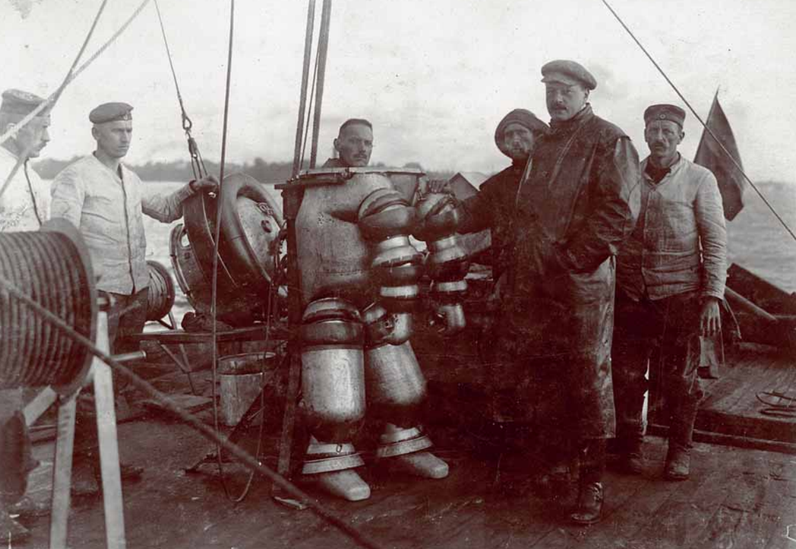
During the world wars salvage operations were particularly risky due to the many mines in the water. This series of photos shows a diver testing an armoured diving suit presumably during the First World War.
